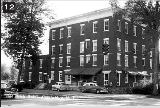
In the 1950s, Joe Powers ran the barbershop in the addition of the Red Brick Hotel (left). Note the upper of the two small windows above the dark awning in the middle of the photograph. Unlike the other windows, this one is dark. According to local folklore, it was a fake window disguising a hidden passage at the end of the hallway.
